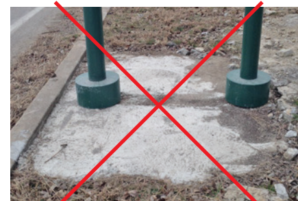
NOT Acceptable Footer Detail
