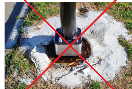
NOT Acceptable Footer Detail
