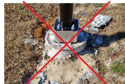
NOT Acceptable Footer Detail
