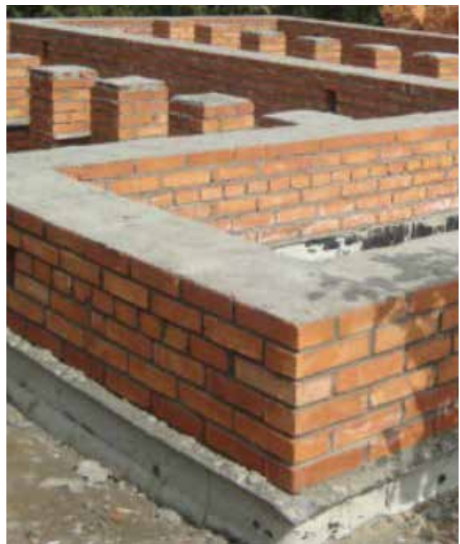
Masonry work at Willis Johnson House
