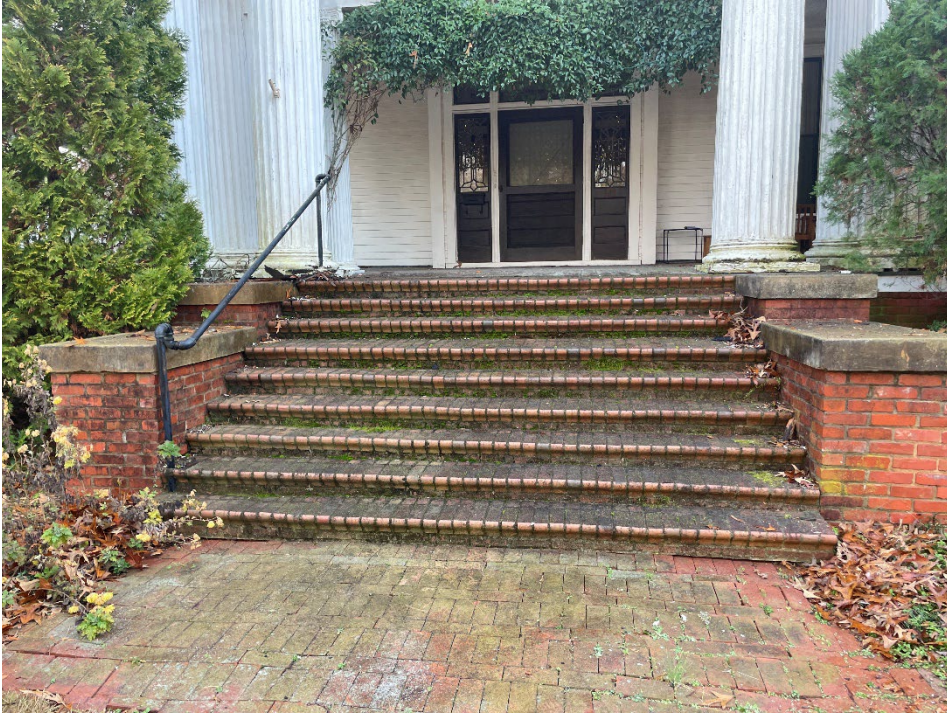
Photo 1: Brick front porch stairs and shoulders.
