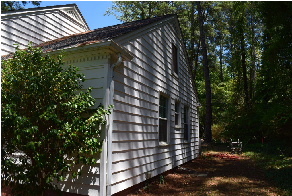
Photo 3: Southwest corner (south elevation)
