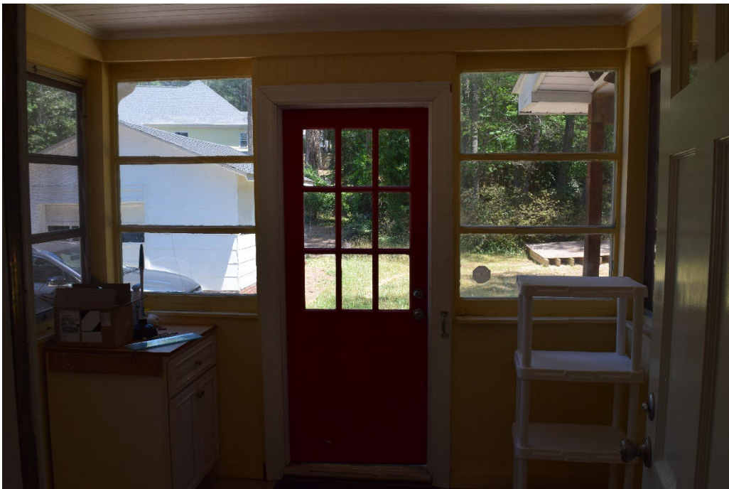
Photo 4: Rear porch facing east.
