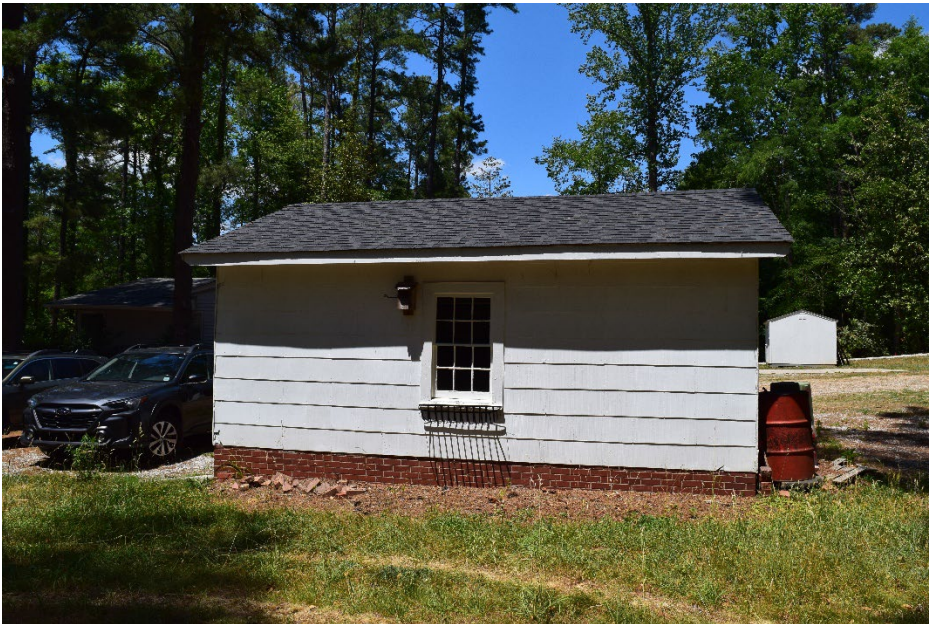
Photo 12: Detached garage facing north.
