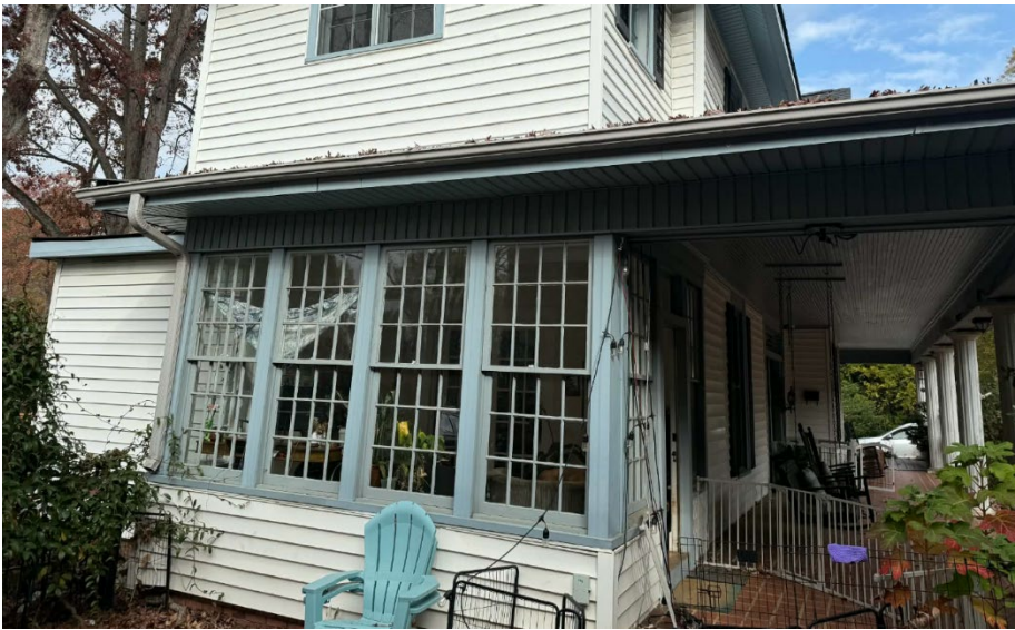
Photo 9: Existing gutters along the south elevation of the porch.
