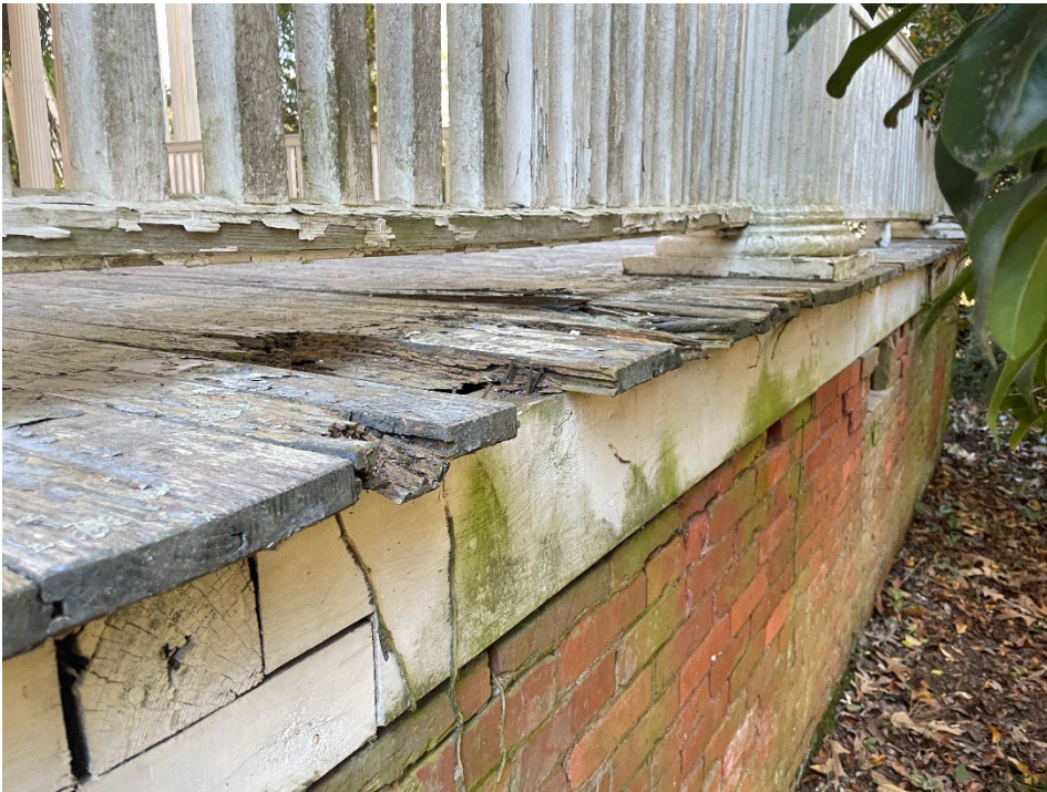
Photo 2: Deteriorated porch decking.
