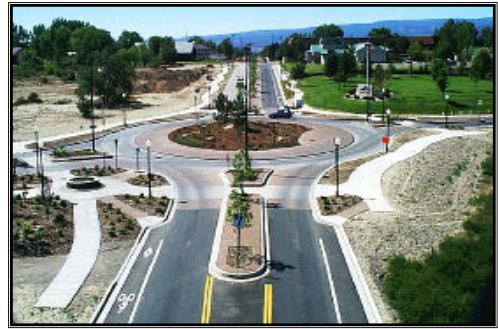
Photo 16: Roundabouts with Bike Lane
