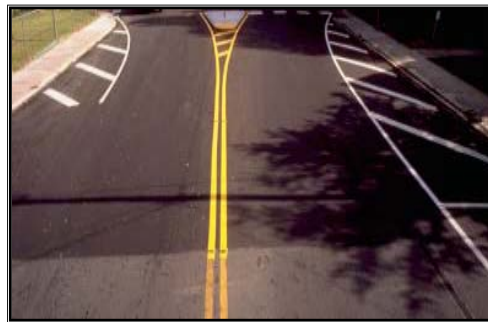
Photo 4: Pavement Markings to visually narrow travel lanes
