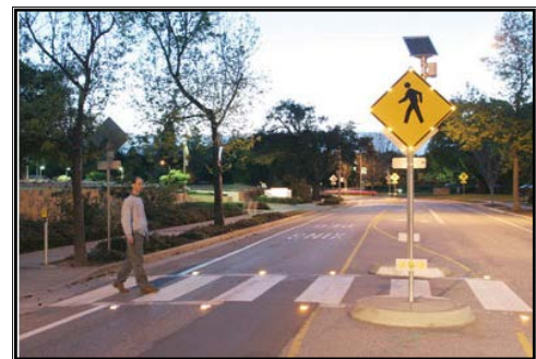
Photo 10: High Visibility Crosswalks
