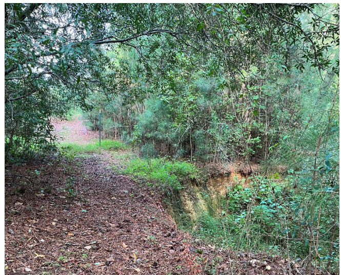
Erosion at dam in the Fairlake neighborhood, identified as a stakeholder concern.
