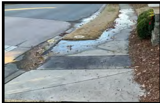
Photo 4: Location: Flemming House St
