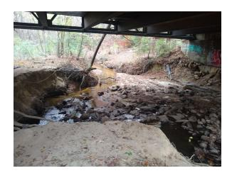
Figure 11. Severe Erosion on Toms Creek
